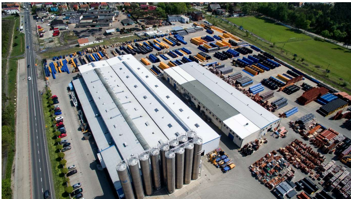
Figure 1. Production plant in Piaski.
